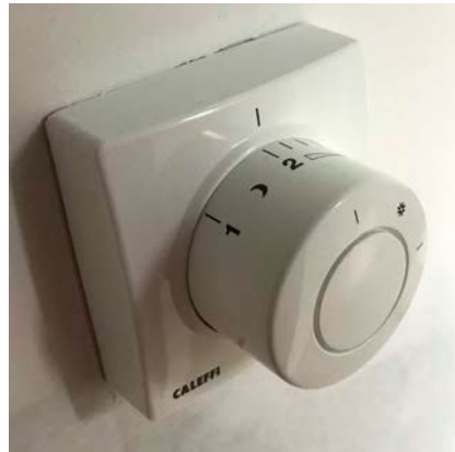
Figure 1: This wall-mounted knob acts like a non-electric thermostatic valve on a radiator.
